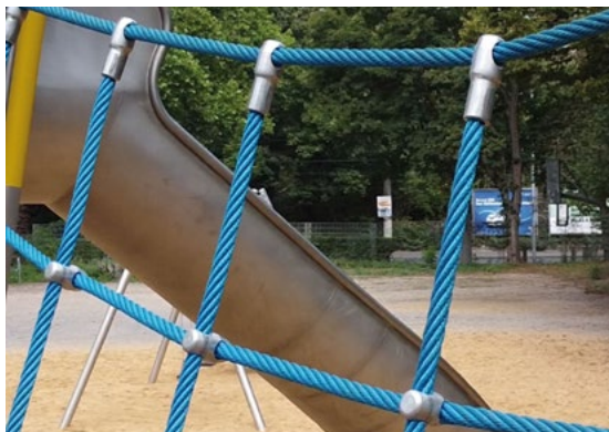
Aluminum connectors for fixation of ropes and large-meshed nets
