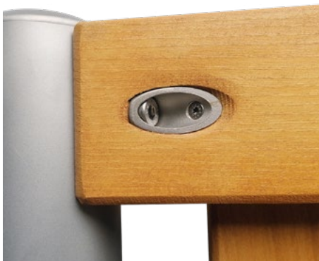
Stainless steel cover on balustrades to avoid drying cracks
