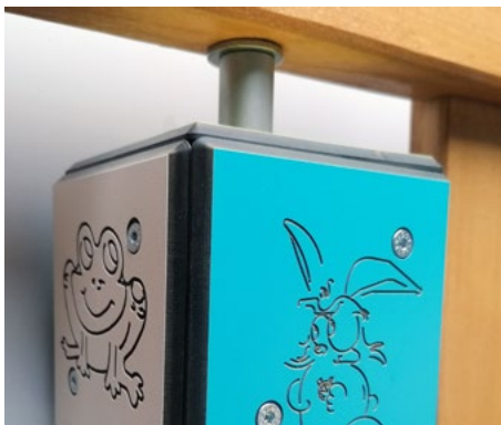
Stainless steel bearings of effect rotating cubes on balustrades
