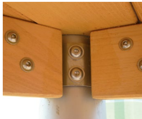
Hidden connection from platform and support posts
