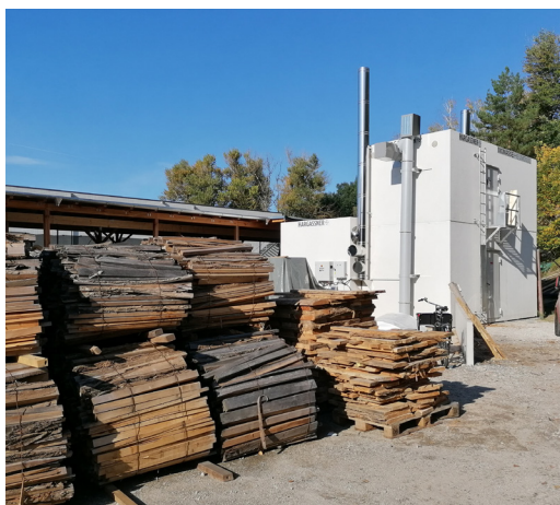
Heat supply by heating with wood waste
