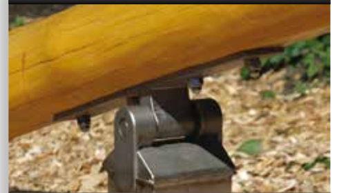
DETAIL: STAINLESS STEEL WIPED BEARING
