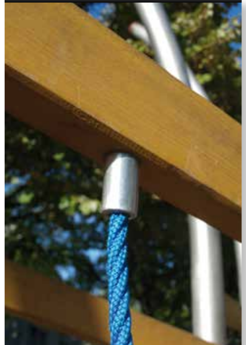
CONNECTION ROPE TO BALUSTRADE
