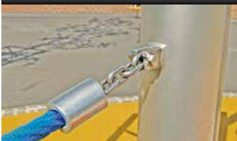
CONNECTION ROPE AND POST
