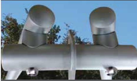
DETAIL: CABLE SLIDE
