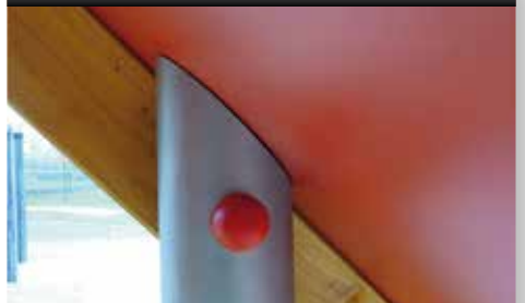
CONNECTION HPL SADDLE ROOF
