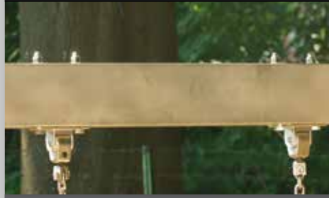
SWING PIVOT POINTS - STAINLESS STEEL
