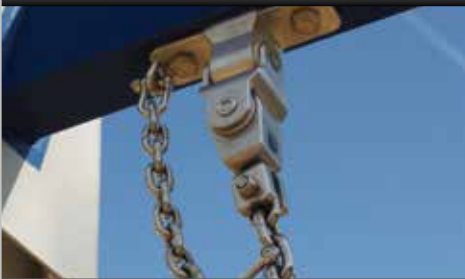
NEST SWING JOINT / ARRESTING CHAIN
