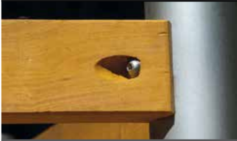
CONNECTION BALUSTRADE TO POST
